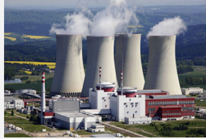
Task fig.3 – Nuclear power station Temelin, Czech Republic
