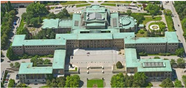
Fig. 7. Parliament TBMM building by Clemens Holzmeister
