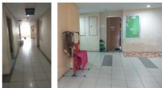
Fig. 14. Seating did not Provided at Flats Corridors.
