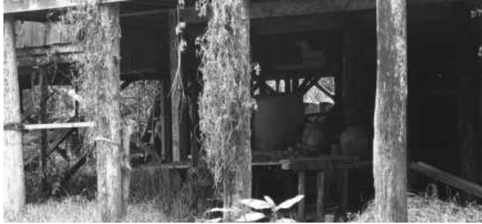
Fig. 4. Solid Belian Tree Trunks as Columns
