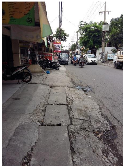
Fig. 3. The accessible pathway were found nearby the PCU Main Campus, but there was no curb ramps and no stable, firm, and slip-resistant walking surfaces. The non PwDs could access but PwDs would find difficulties.
