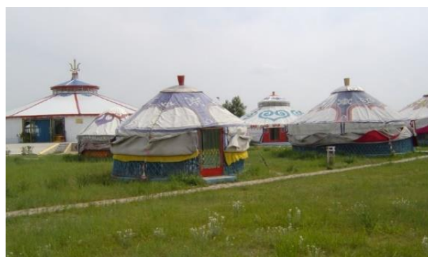
Fig. 3. Ethnographic facility in the Duerbote-Mongol Autonomous region, Heilongjiang Province, China (author's photo)
