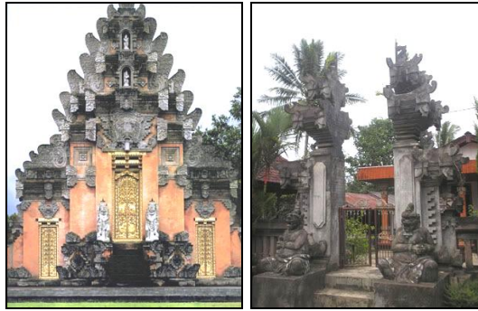
Fig. 11. Entrance gate ( Candi Bentar & Kori ) in Balinese traditional building (Personal Documentation, 2005).
