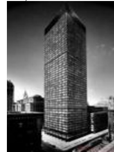
Fig.5 Union Carbonized Building
