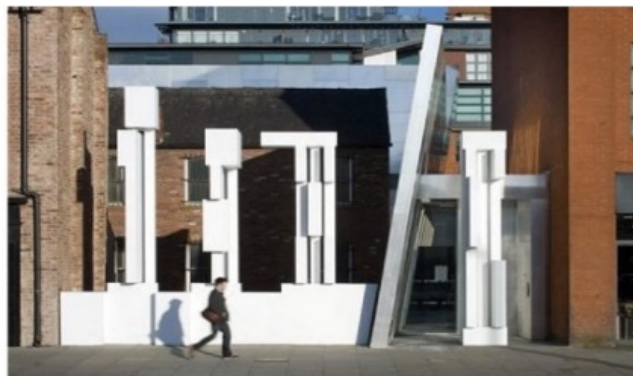
The front of the building
